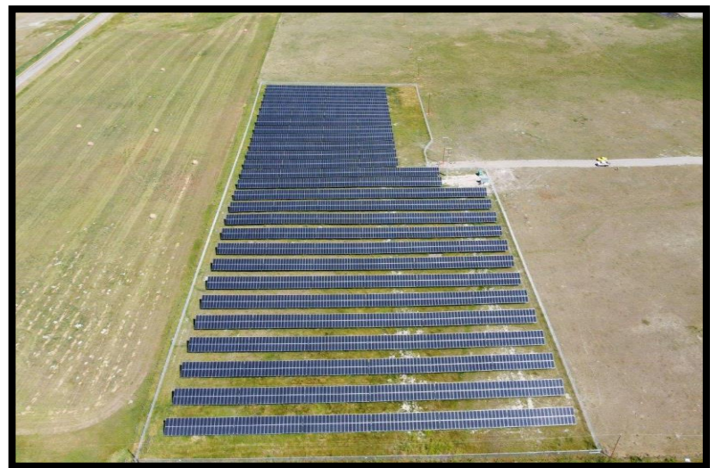
TOWN OF CARDSTON SOLAR PARK
